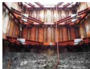
Construction method for waterproof walls between tubular piles based on the Gyopress Method™
